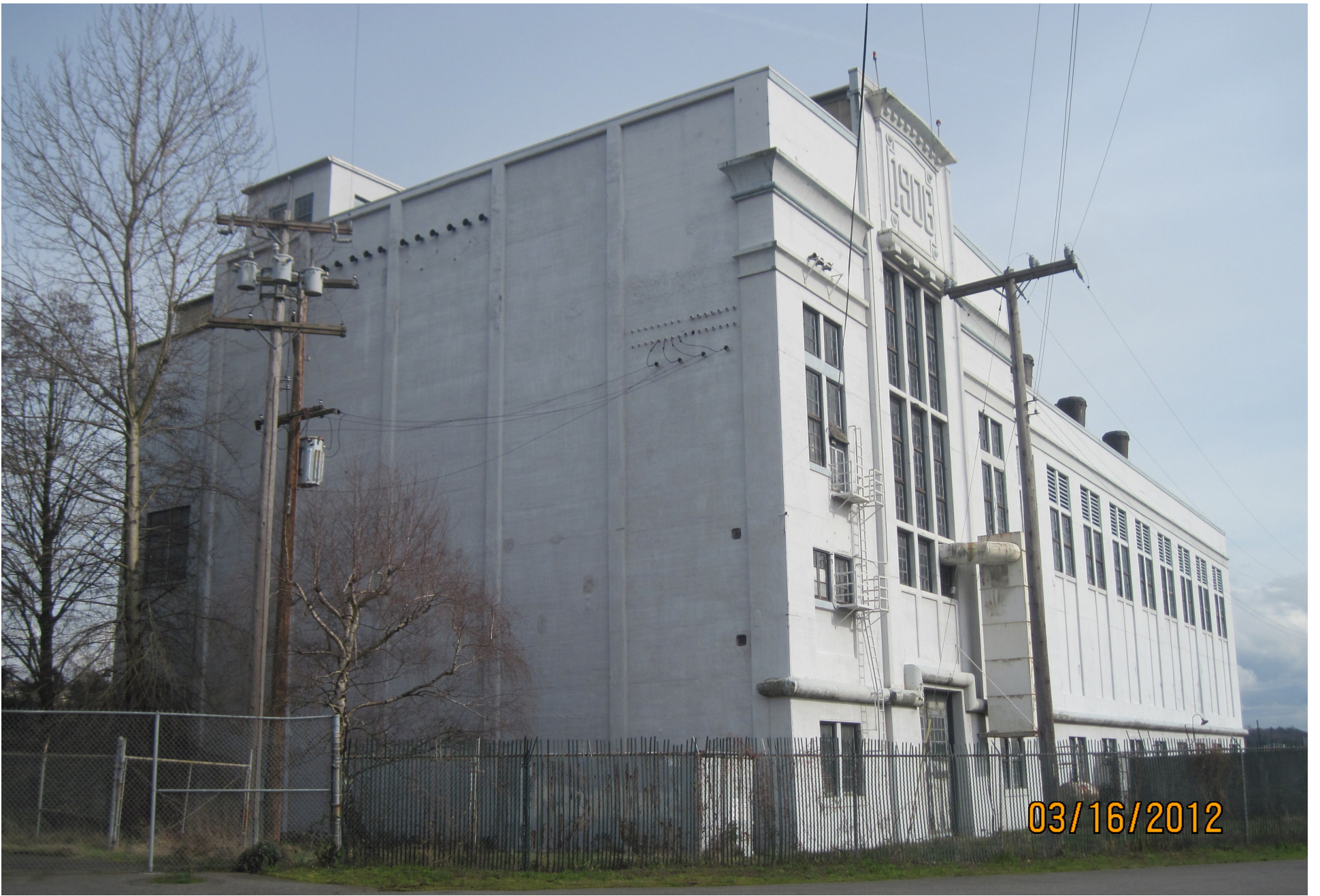
1. EXTERIOR LOOKING SOUTHEAST
