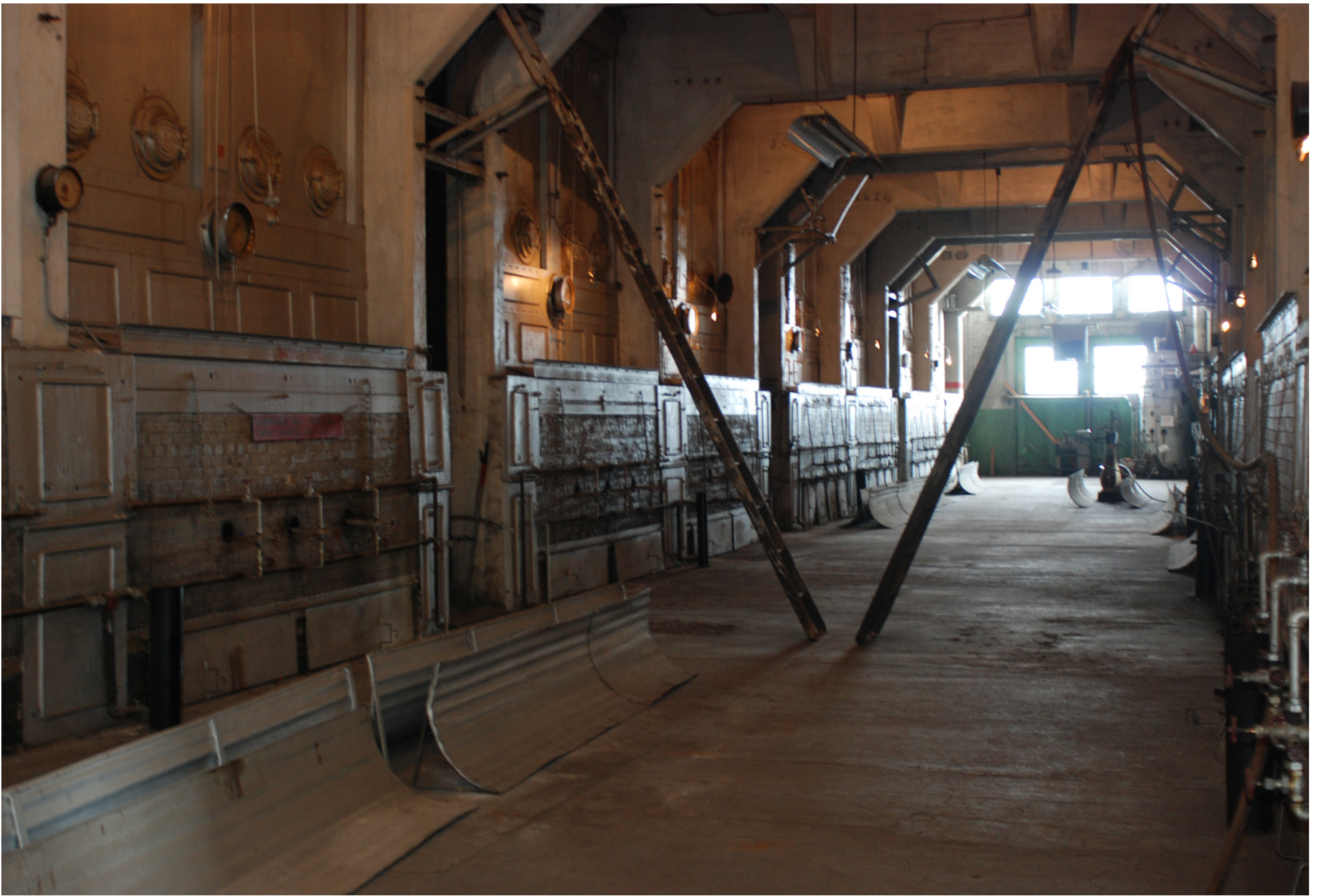
3. BOILER ROOM LOOKING SOUTH
