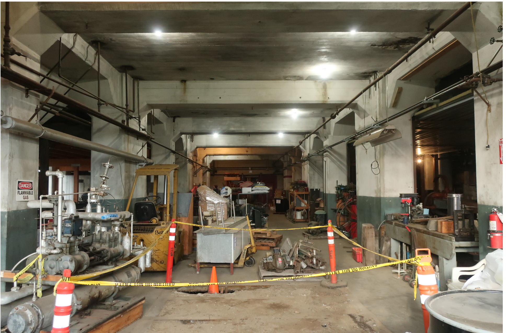
4. ASH ROOM LOOKING NORTH
