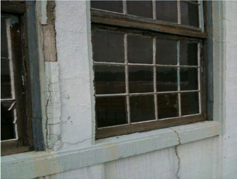
Photograph 5. HSA 2: Grey/white window putty glazing (M)
