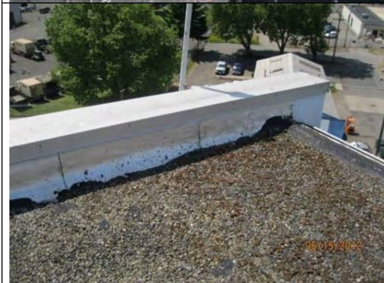
Photograph 13: West end of upper roof with raised parapet.
