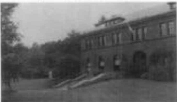
(d.) Harnswell Visitor's Center's entrance following rehabilitation, integrating an accessible path (left), platform, and new steps. Photo: Charles Birdman.
