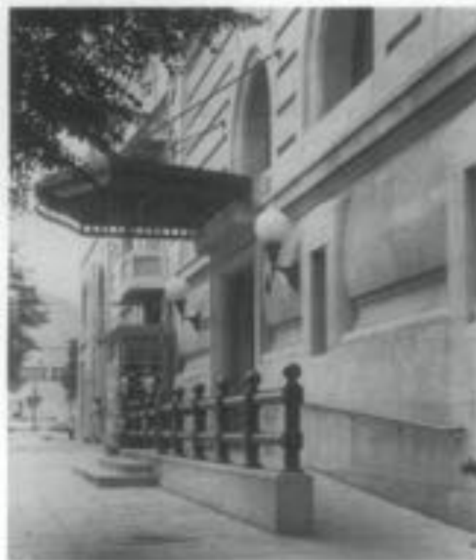
Figure 9. This ramp was created by infilling the window-well and slightly modifying the historic railing. The ramp preserves this building's historic character. Photo: Thomas Jester.
