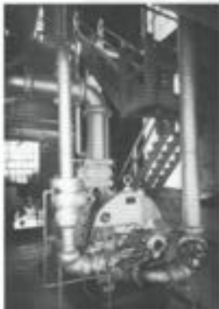
1917 average distribution steam turbine being fed by horizontal turbine steam turbine.
