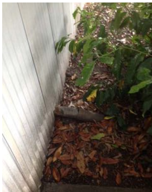
Image 6: East side Boiler Rm drain pipe
