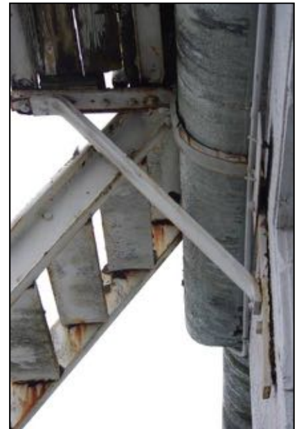
Figure 1-7: South Fire Escape, Detail
