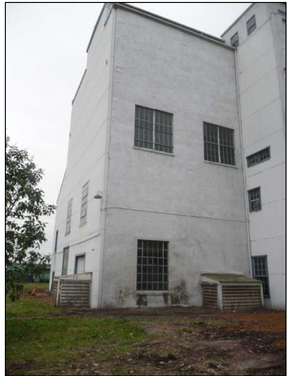
Figure 62: Looking southwest toward the north wall of the 1918 Addition, with stucco-clad hollow clay tile.
