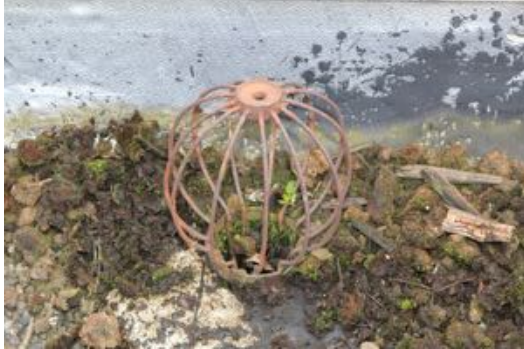
Image 1: Existing roof drain
