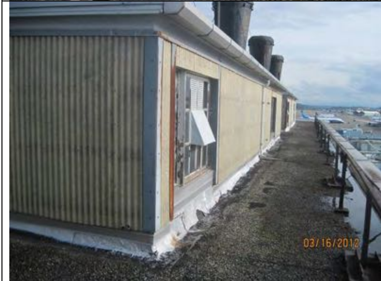
Photograph 21: Looking south along west edge of southern roof area.
