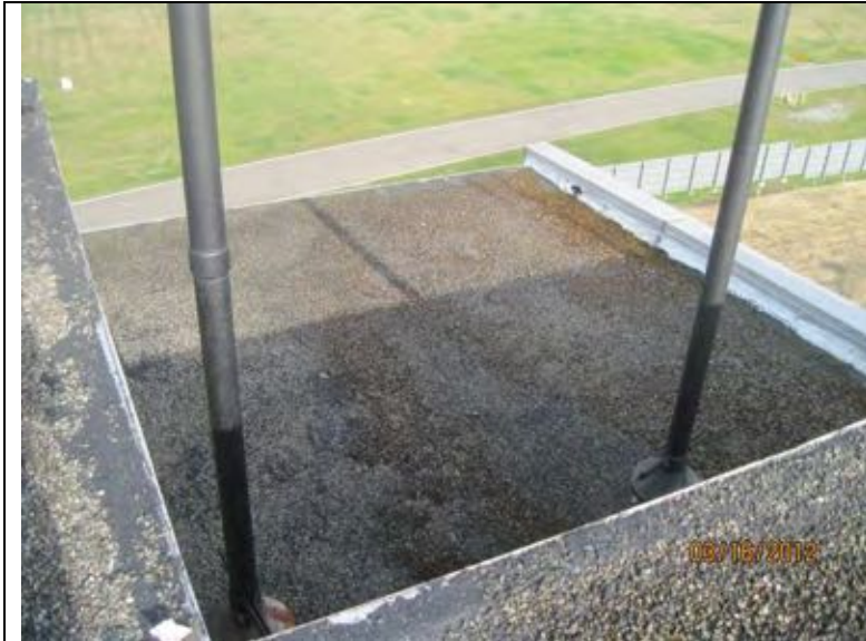
Photograph 20: Low SE roof.
