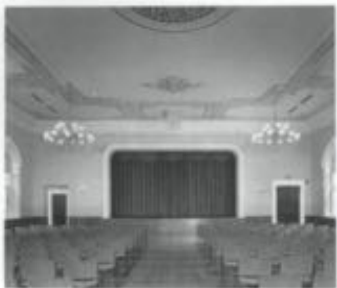
9. Town Hall, Andover, MA. The upstairs auditorium was restored and new mechanical systems were installed. Perimeter baseboard radiative heat and air handlers, located in the attic space provide air conditioning. The cast iron ceiling grille was adapted for return air and the supply registers were installed in a symmetrical and regular manner to minimize impact on the historic ceiling. Photo: David Hewitt/Anna Garrison for Ann Beha Associates.
