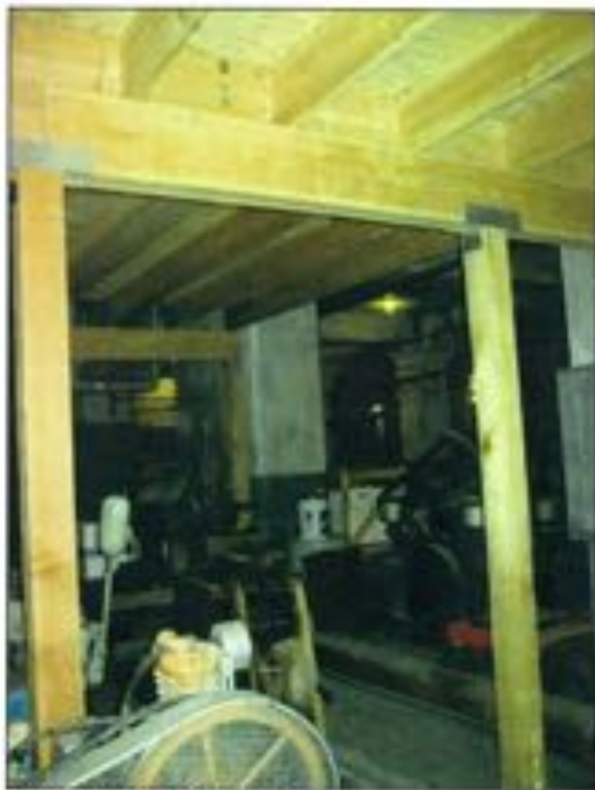
Figure 1-5: Wood platform on west bay.
