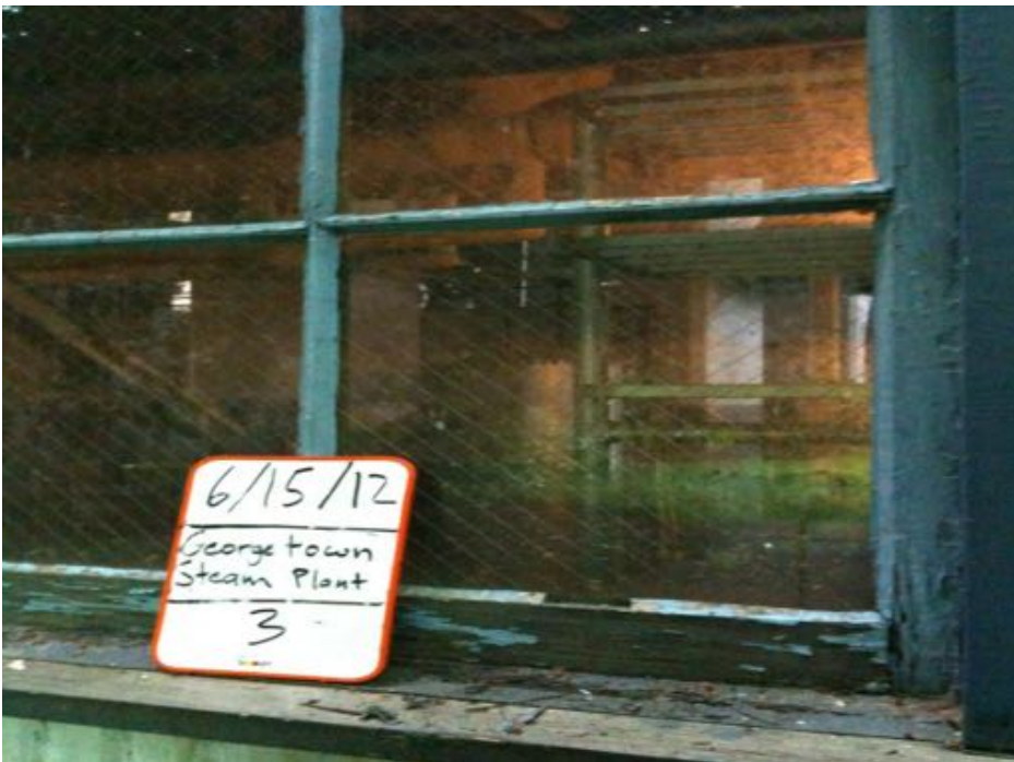
Photograph 6. HSA 3: White window putty glazing with paint (M)
