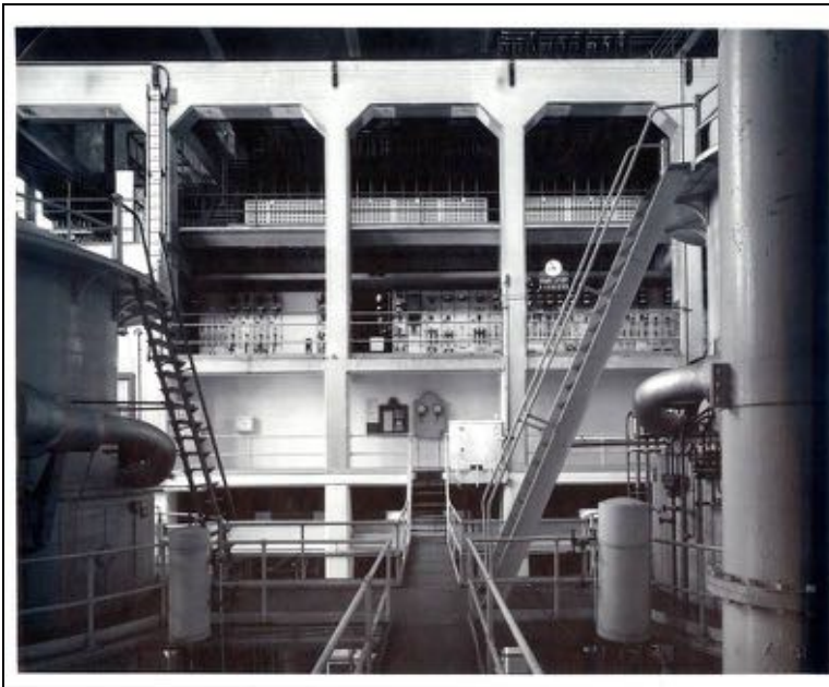
View looking north toward the Boiler Room galleries. (HAER, 1984)
