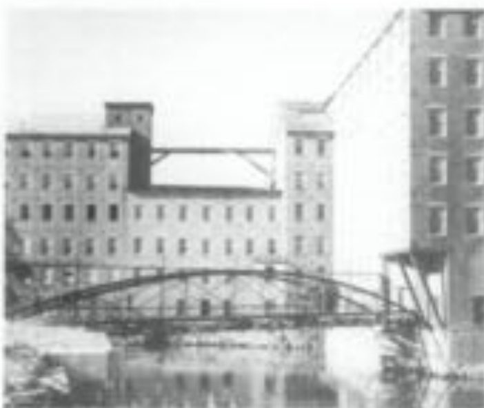
Figure 1. Windows are frequently important visual focal points, especially on simple facades such as this mill building. Replacement of the multi-pane windows here with larger panes could dramatically change the appearance of the building. The areas of missing windows convey the impression of such a change. Photo: John F. Lenz
