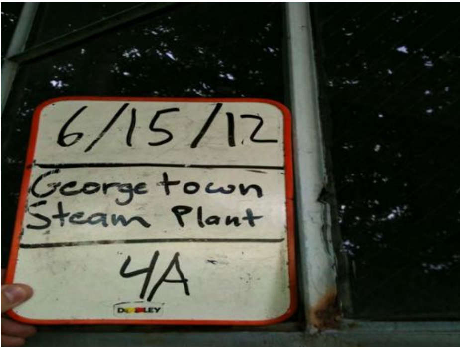
Photograph 8. HSA 4A: Black sealant with paint (M)
