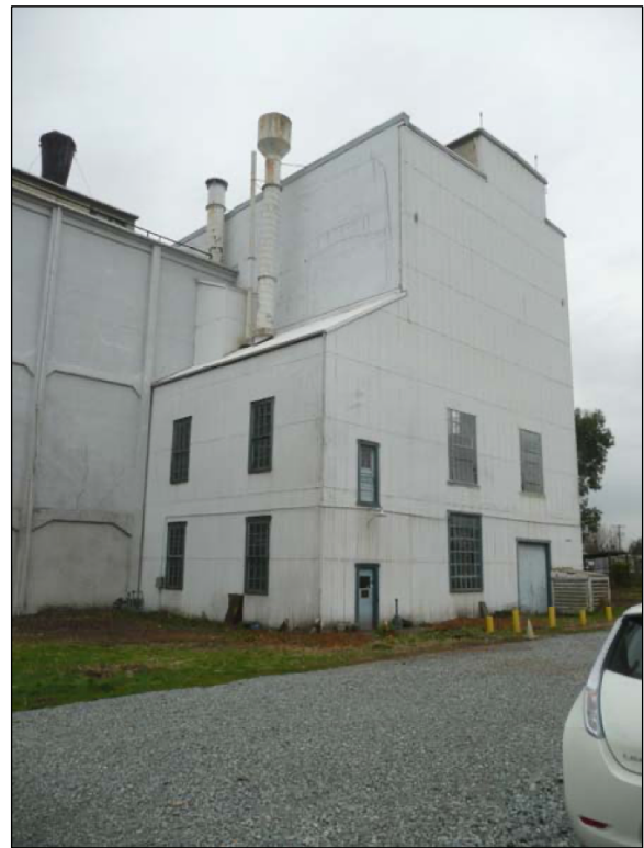
Figure 59: East and south walls of the 1918 Addition with corrugated metal cladding.
