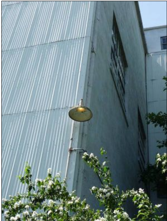
Figure 83: Exterior light at the northeast corner of the 1918 Addition, which is on in the middle of the day.
