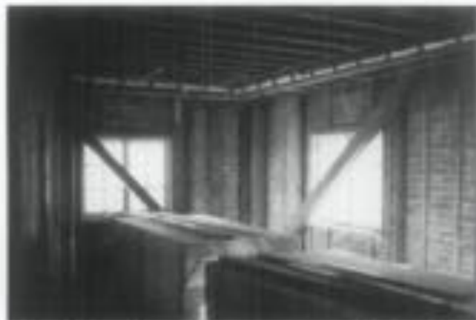
2. Standard approaches to seismic retrofit, as seen with the diagonally braced frame crossing in front of the historic windows, are visually intrusive. Solutions, such as using hidden moment frames around the perimeter of the windows, will meet the goals of historic preservation and seismic retrofit. Photos: Strand Design.
