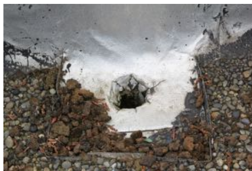
Image 4: Existing roof drain
