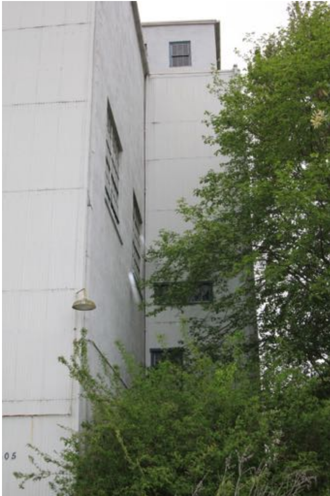
Image 10: Exterior Light Fixture
