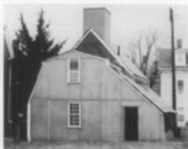
Temporary stabilization or "mushbelling" with materials such as plywood and building paper can protect the roof of a project until it can be properly repaired or replaced. (Narbonne House, Salem, Massachusetts)
