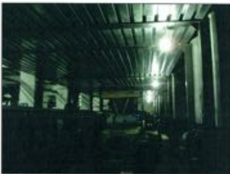
Figure 1-4: Steel platform on east bay.
