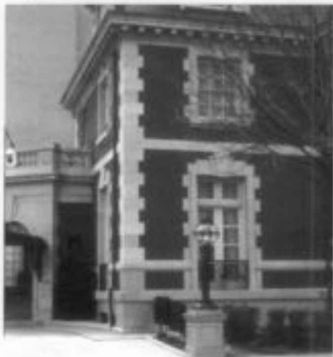
Figure 4. The foundation of this brick building is limestone, but the decorative trim above is architectural terra cotta intended to simulate stone.
