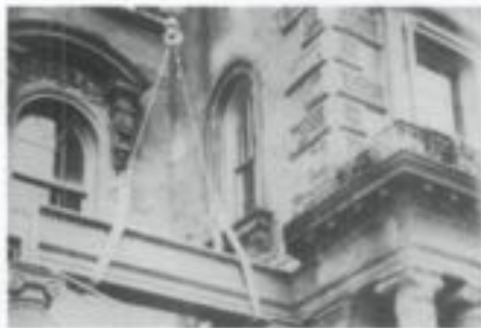
Illus. 8. Simple solutions should not be overlooked when materials are no longer available. In the case of the Morse-Libby Mansion (1838), Portland, ME, the deteriorated ironstone porch beam was replaced with a carved wooden beam painted with sand impregnated paint. Photo: Stephen Sewall.
