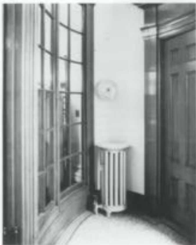
6. A condition assessment during the planning stage would identify this ornate radiator in a small oval-shaped niche as a significant element of the historic heating system. In upgrading the mechanical system, the radiator should be retained. Photo: Michael C. Hovig, P.E., AIA.
