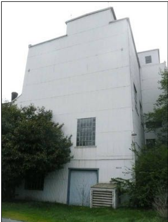
Figure 58: East wall of the 1918 Addition with corrugated metal cladding.
