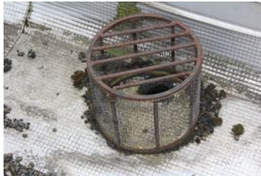
Image 2: Existing roof drain
