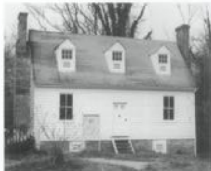
Figure 10. Regrading around the Tucker Troncent at Colonial Williamsburg has protected the masonry foundation soil from excessive damp. This building has been successfully mothballed for over 20 years. Note the attic and basement vents, the temporary stairs, and the information sign interpreting the history of this building.
