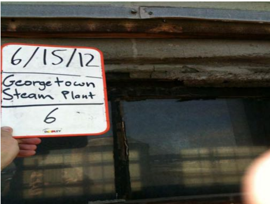
Photograph 10. HSA 6: Grey cementitious material and black asphaltic material (S)
