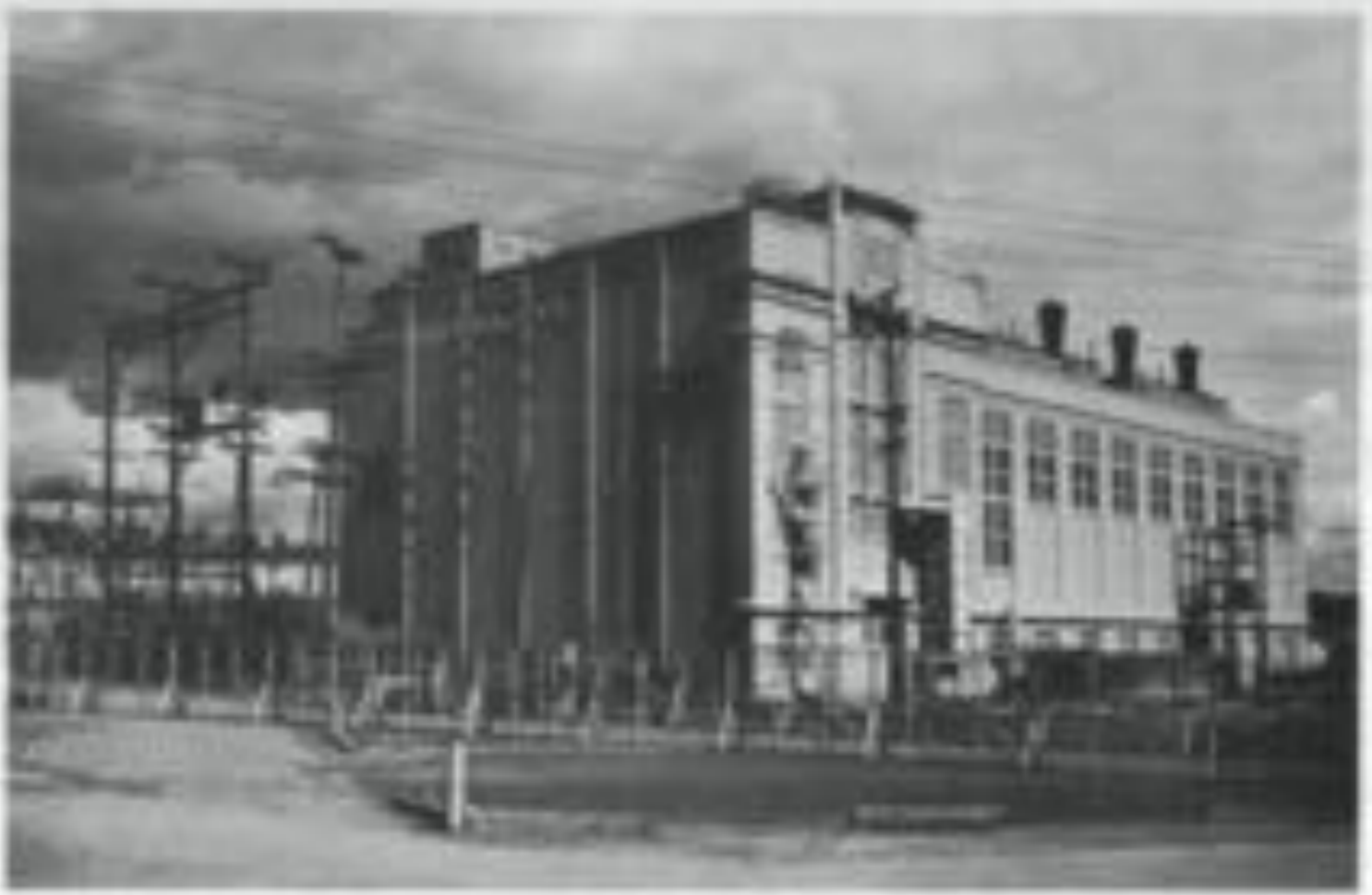
LANGSTON STEAM PLANT SEATTLE, WASHINGTON
