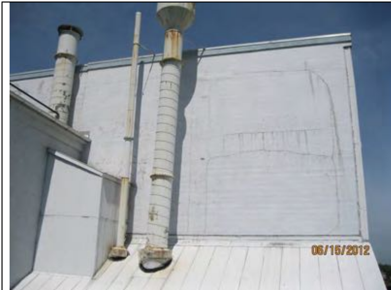
Photo 29: South facing wall at engine room addition. Corrugated metal roofing below.
