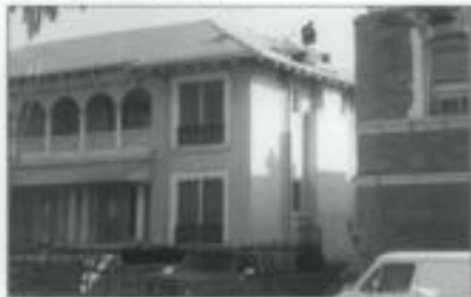
4. The compact size and good condition of the masonry building on the left withstood the earthquake except for the loss of the unsupported chimney at the roof line. The brick building on the right appears to have sustained more damage. Photo: Steve Crisp.
