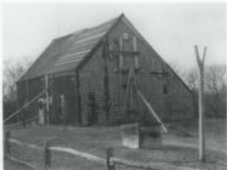
Figure 3. Buildings seriously damaged by storms or deterioration may need to be shored before architectural evaluations can be made. Joffin Coffin House. Photo: John Miller Architects.
