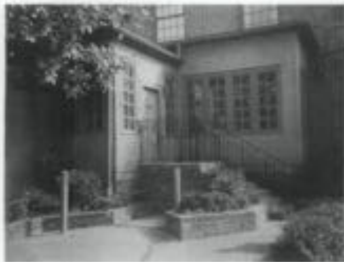
Figure 14. At the Lieutenant Governor's Mansion in Frankfort, Kentucky, a retracting lift (R) was installed to minimize the visual effect on this historic building when not in use (L). Photo: Aging Technology Incorporated.
