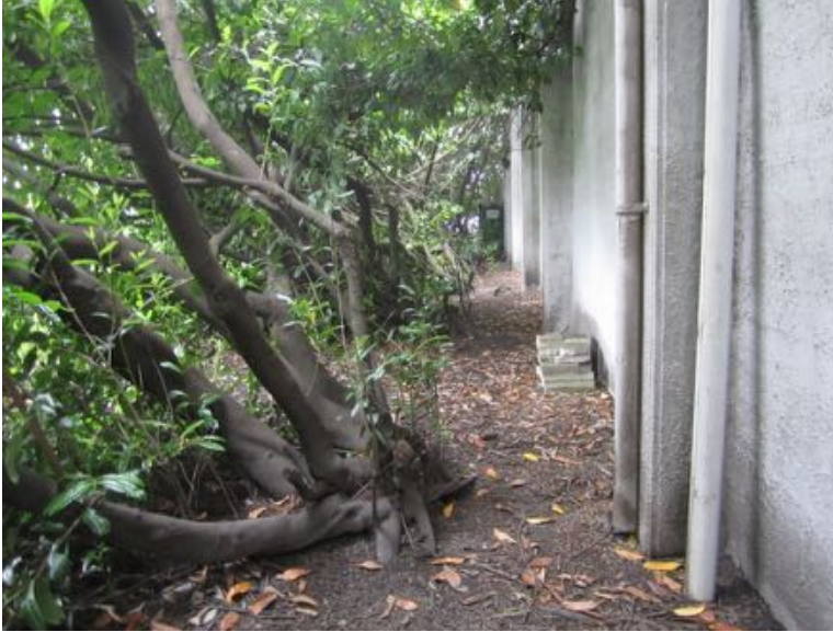
Figure 43: View south along the east façade, showing the extent of Laurels. (KKLA)
