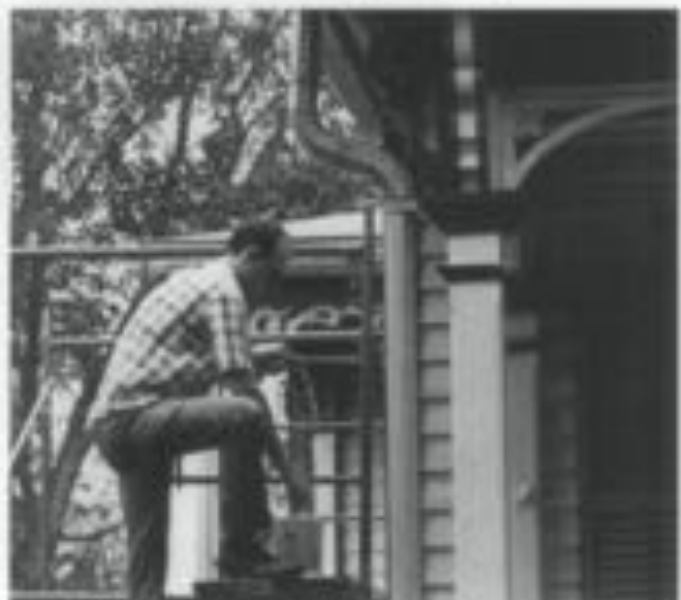
Fig. 19. Maintaining gutters and downspouts in good operable condition, requiring eaves to keep water out, redirecting damaging moisture away from foundations and controlling interior moisture and condensation are all important when holding the line on moisture deterioration. Photo: Nebraska State Historical Society.
