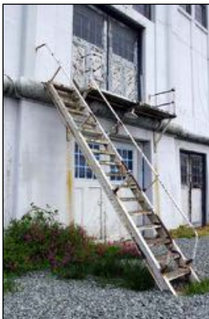
Figure 1-3: South Fire Escape
