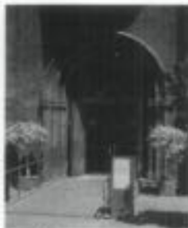
Figure 12. The Smithsonian Institution installed a temporary ramp on its visitor's center to allow adequate time to design an appropriate permanent ramp. Photo: Thomas Jester.
