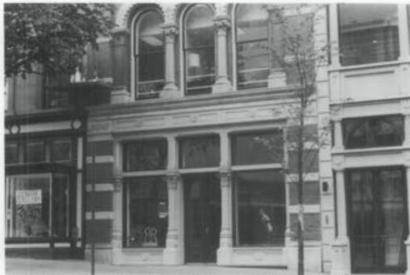
The new cast aluminum storefront replaced the last 19th-century cast-iron original. Photo: Sharon C. Park, AIA.
