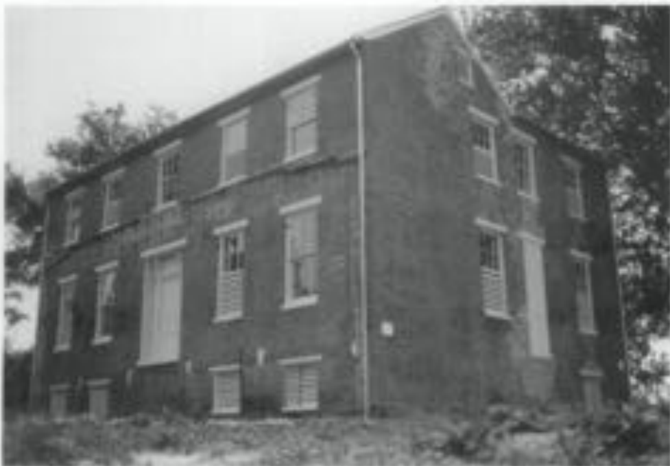
Figure 1. Proper mothballing treatment: This building has been successfully mothballed for 10 years because the roof and walls were repaired and structurally stabilized, ventilative louvers were added, and the property is maintained. Photo: Charles E. Fisher, NPS.
