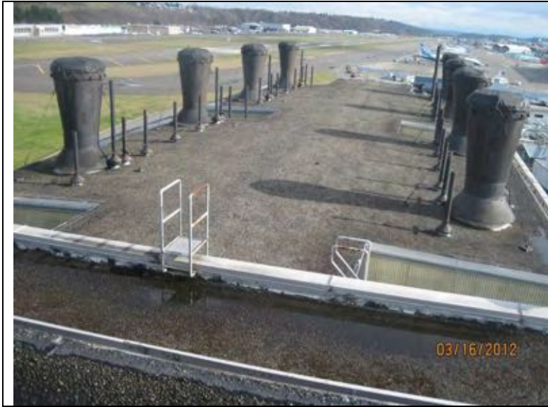
Photograph 14: Looking south from the upper north roof.
