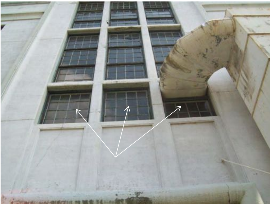
Photograph 16. HSA 12: Window putty glazing with 4 by 4 window pane pattern (M)
