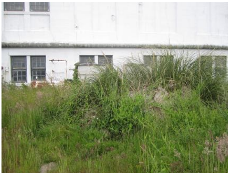
Figure 45: View of Pampas Grass, west yard. (KKLA)
