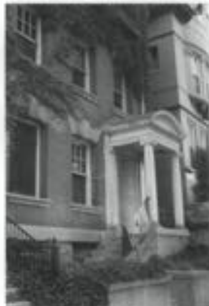
Figure 20. All systems except temporary electric have been shut off as the maintenance effort has been restricted over 20 years. The electrical meter and 100 amp panel has been been set as a physical guard at the front of the building. It is used for interior lighting and vacuum down systems. The building, however, is showing signs of moisture problems with glass several stories up. The masonry indicating the need for gutter maintenance and additional surveillance for the interior. The negligence of the walls, although permanent, large structure and is damaging to the masonry. Photo by Wood Joint, 2014.
