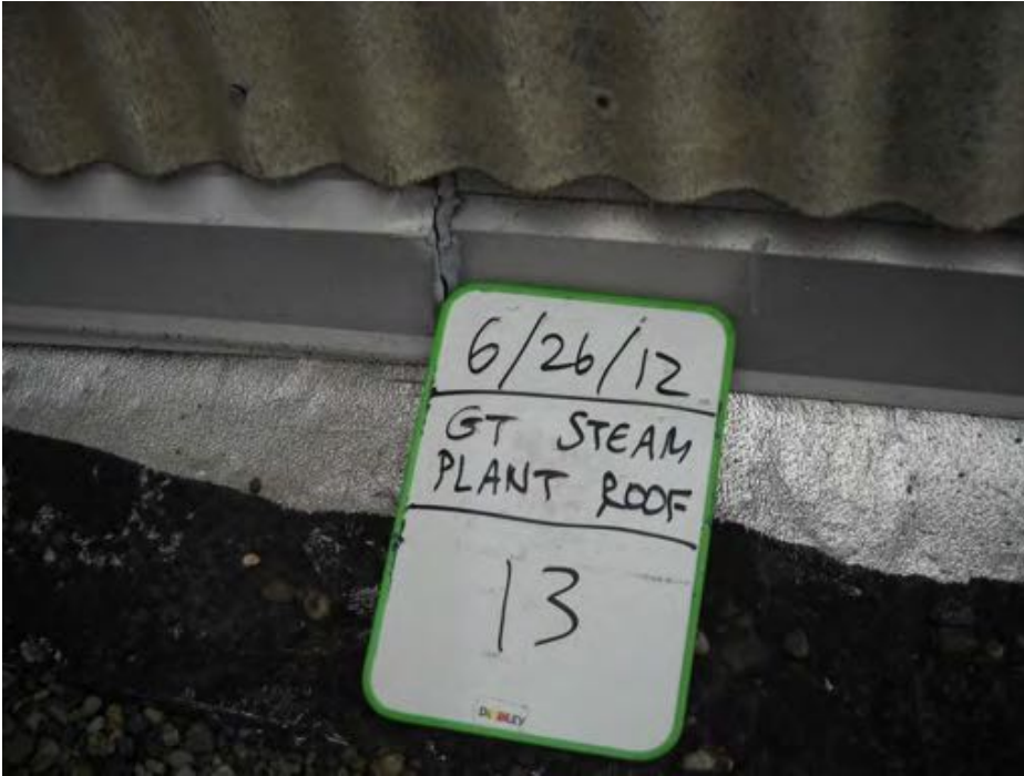
Photograph 13. RF-13: Grey rubber caulking (M)
