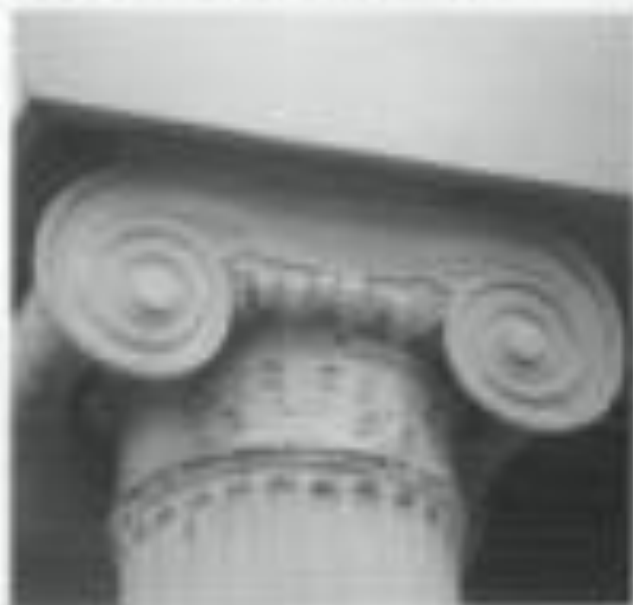
The capital column capital was made using epoxy resin poured into a mold taken from the building. The historic window sashes still are original during the restoration. Photo: George Del Cosentino
