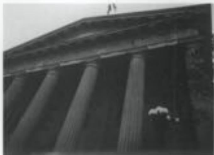
Illus. 13. Code-related changes are of concern in historic preservation projects because the integrity of the historic resource may be irretrievably affected. In the case of the Old San Francisco Mint, the fiberglass cornice was used to bring the building into seismic conformance. The original cornice was deteriorated, and the replacement (1982) was limited to the projecting pediment. The historic stone fascia was retained as were the stone columns. The limited replacement of deteriorated material did not jeopardize the integrity of the building. Photo: Walter M. Southamer.
