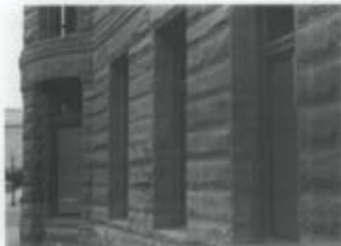
Illus. 16. The good quality substitute materials shown here do match the historic sandstone in color, texture, tooling and surface details. Dry-lump cast stone was used to match the red sandstone that was no longer available. The reconstructed first floor incorporated both historic and substitute materials. Sufficient molds were made to avoid the problem of detecting the substitutes by their uniformity. Photo: Sharon C. Park, AIA.
