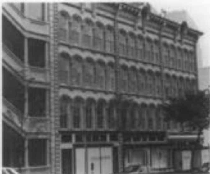
illus. 22. A fiber reinforced polymer (fiberglass) cornice and precast concrete elements replaced deteriorated features on the 19th-century exterior. Photo: Sharon C. Park, AIA.
