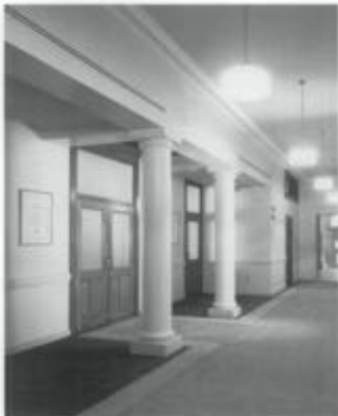
8. Central air conditioning was installed in the corridors of this circa 1900 school building by adding an air handler over the entrance from a rooftop. The custom-designed slot registers provide linear diffusion without detracting from the architecture of the space. Photo: Lautman Photography courtesy of Nitter Finegold + Alexander Inc.
