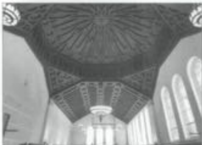
16. During the extensive rehabilitation of this historic building, new concrete, behind the new plaster finishes, strengthened the interior brick walls and additional roof reinforcement was hidden behind the repaired masonry and original ceiling. Photo © Jonathan Ferrer, courtesy UCLA Capital Program.
