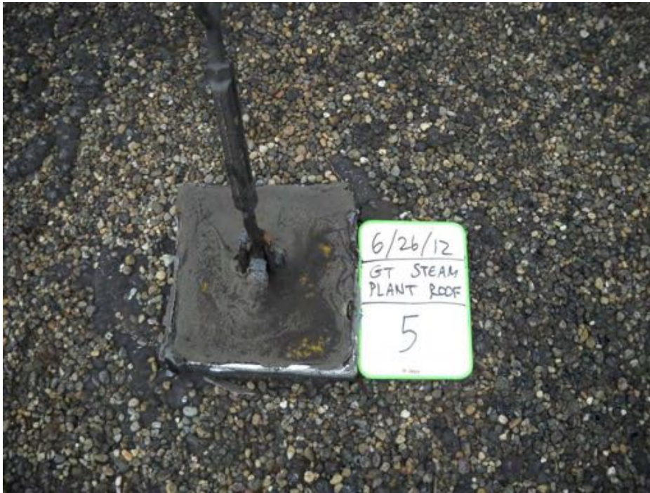
Photograph 5. RF-5: Black asphaltic sealant (M)
