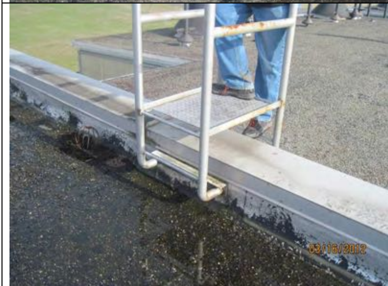
Photograph 16: Ladder to south roofs bolted to interior side of parapet.
