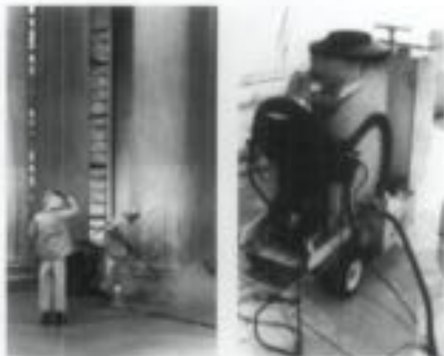
Figure 8. (Left) Low-pressure (under 100 psi) steam cleaning (hot pressurized water washing), is part of the regular maintenance program at the Jefferson Memorial, Washington, D.C. The white marble interior of this open structure is subject to constant soiling by birds, insects and visitors. (Right) This portable steam cleaner enables prompt cleanup when necessary. Photos: National Park Service files.
