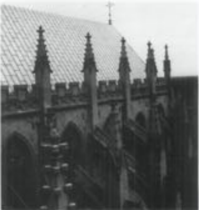
Good design and quality materials for the roof surface, framings, and flashing minimize roofing failures. This is essential on roofs such as on the National Cathedral where a thorough maintenance inspection and minor repairs cannot be done easily without special roof jacking. Moreover, the success of the roof on any structure depends on frequent cleaning and repair of the gutter system. (Washington, D.C., photo courtesy of John Burns, A.I.A.)
