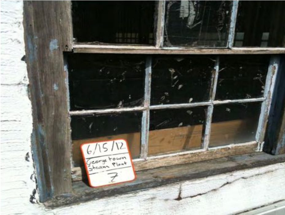
Photograph 11. HSA 7: White/grey window putty glazing (M)
