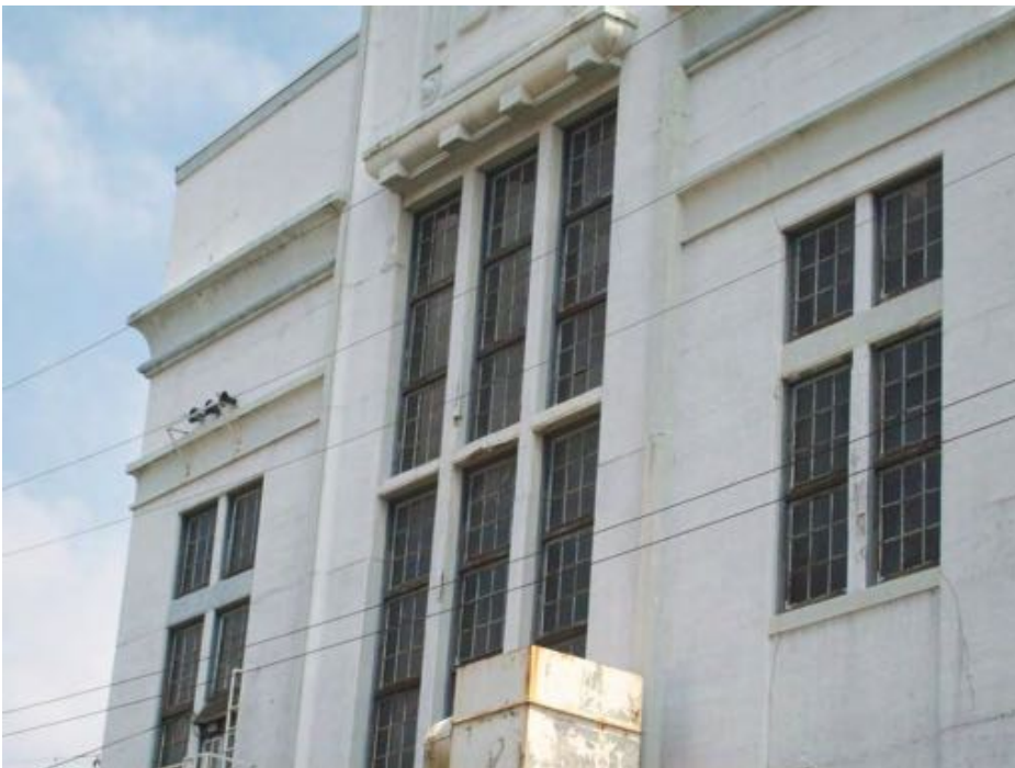
Photograph 14. HSA 10: Window putty glazing with 4 by 3 window pane pattern (M)
