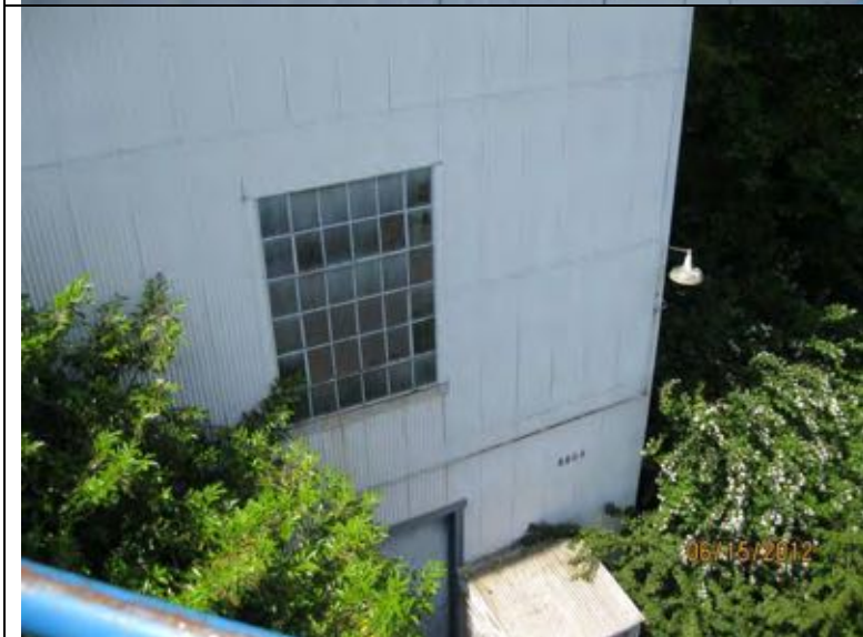
Photo 53: Overview of east wall of engine room, 1918 addition. Steel framed windows are present.
