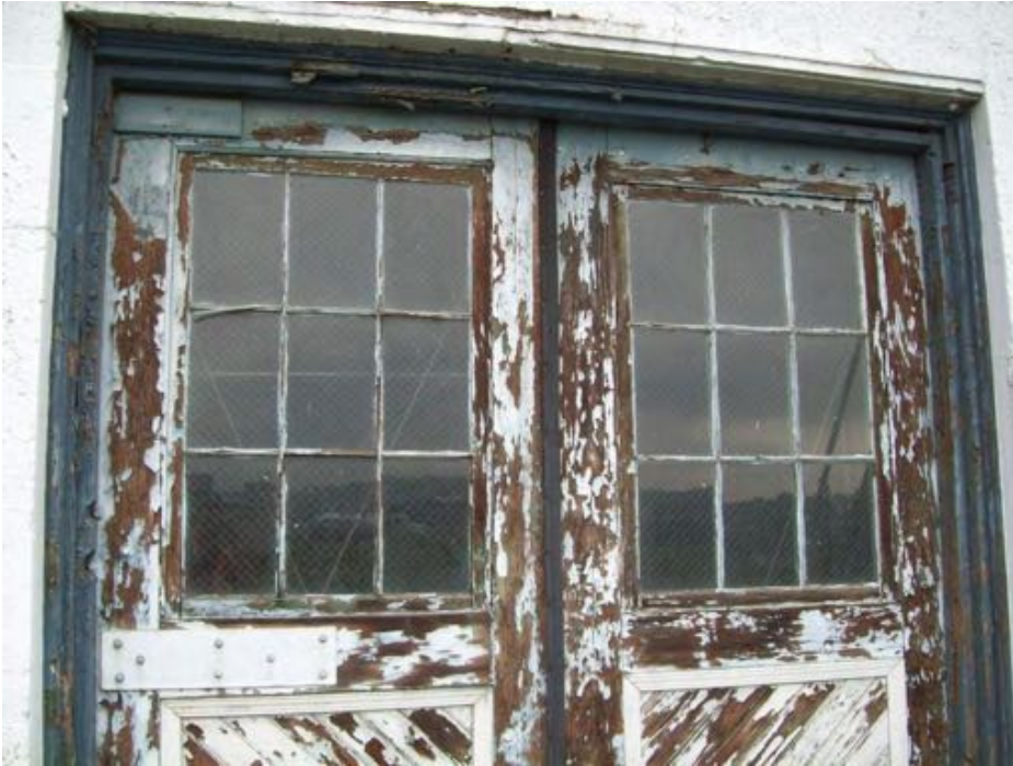
Photograph 9. HSA 5: Off-white window putty glazing with paint (M)
