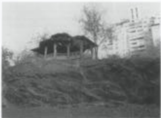
Figure 35-37: Central Park has developed an in-house historic preservation crew to undertake small projects. A specialized crew has been trained to specifically repair and rebuild rustic furnishings. As illustrated, the restoration of the Dewey rustic shelter was achieved by constructing it in the Ramble compound, moving it in place opposite 67th Street and completed. Courtesy Central Park Conservancy.
