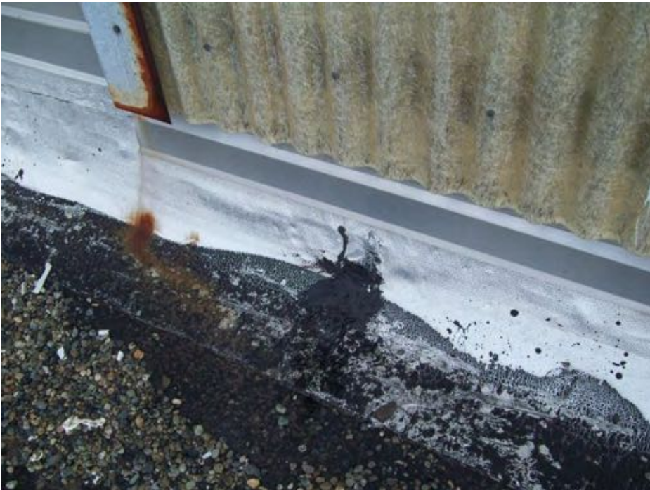
Photograph 18. RF-18: Silver foil over black built-up roofing over black felt (M)
