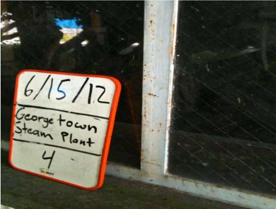
Photograph 7. HSA 4: Grey window putty glazing and black brittle material (M)
