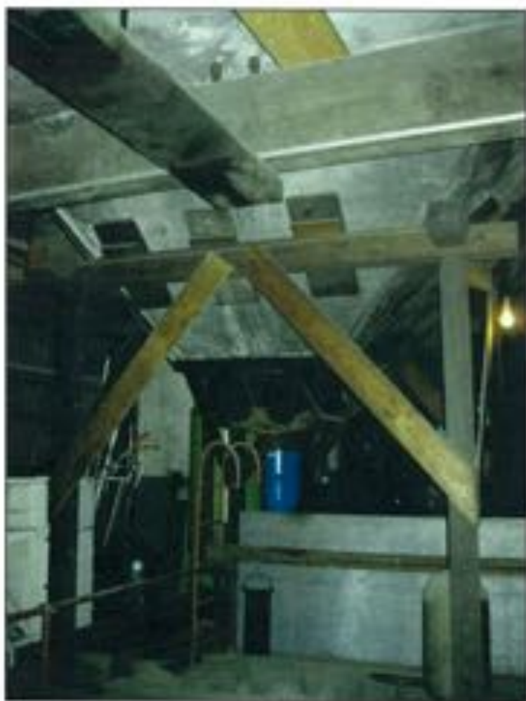
Figure 1-6: Timber shoring of intact ash hopper
