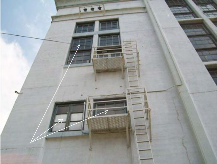
Photograph 15. HSA 11: Window putty glazing with 3 by 3 window pane pattern (M)
