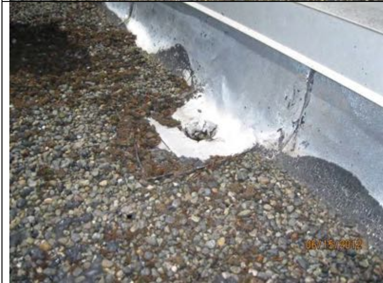
Photograph 4: Typical drop drain adjacent raised perimeter edges.
