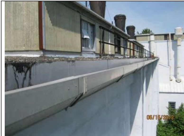
Photo 26: Gutter on east side of south roof area.
