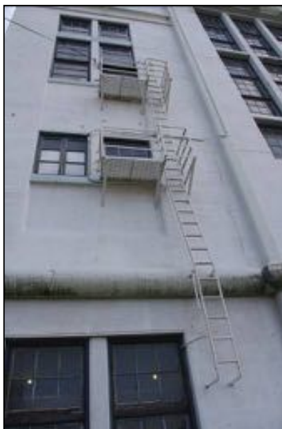
Figure 1-2: Northwest Fire Escape
