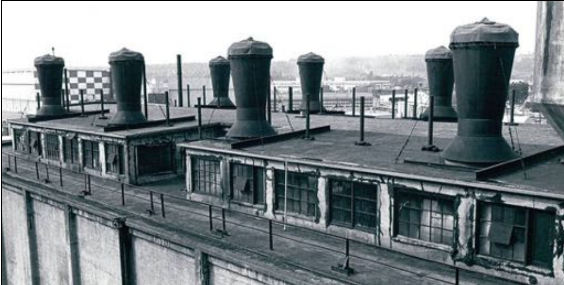
Figure 56: This undated photo shows an example of the extent of repairs to the monitor walls and windows prior to the installation of the fiberglass panels. (Photo courtesy of SCL)
