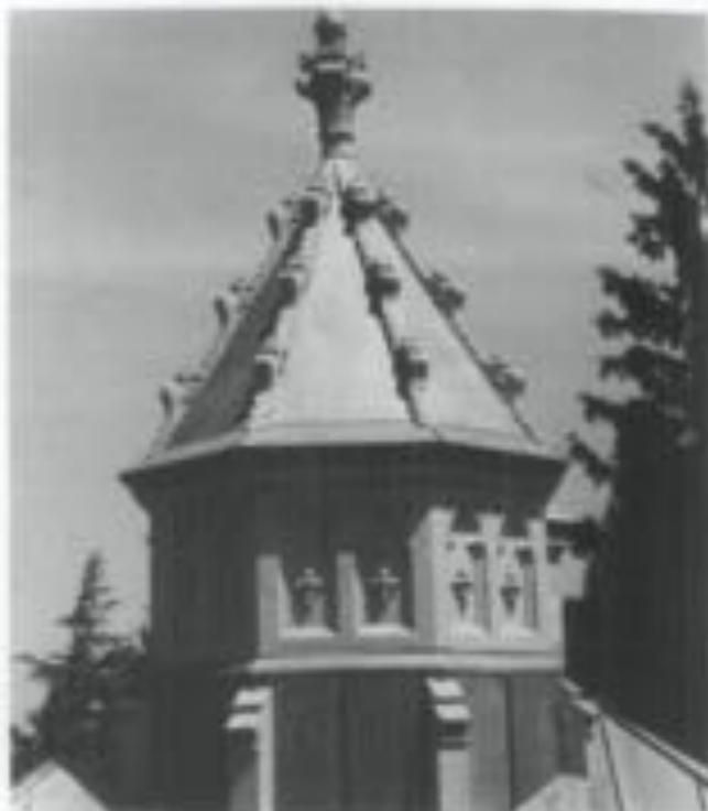
Decorative features such as cupolas require extra maintenance. The flashing is carefully detailed to promote run-off, and the wooden ribbing must be kept well-painted. This roof surface, which was originally tin plate, has been replaced with lead-coated copper for maintenance purposes. (Lyndhurst, Tarrytown, New York, photo courtesy of the National Trust for Historic Preservation)
