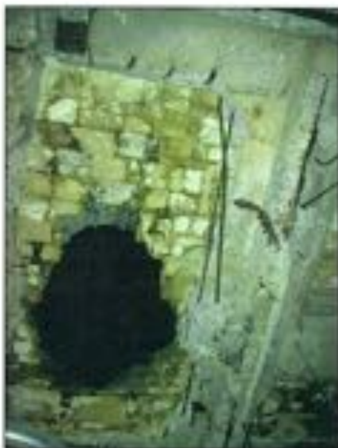
Figure 1-3: Partially demolished ash hopper viewed from below.
