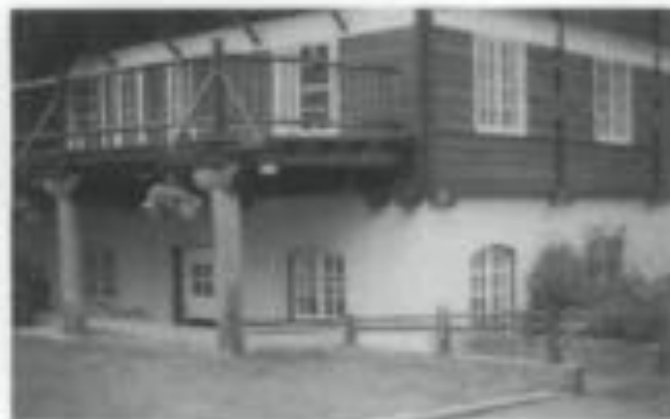
Figure 8. A new below-grade ramp provides access to Lake MacDonnell Lodge in Glacier National Park. Photo: Thomas Jester
