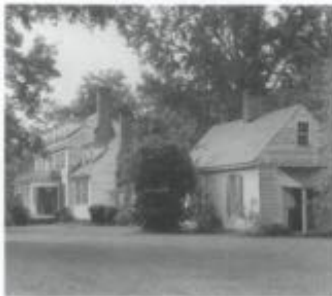
1. Eighteenth century and later vernacular architecture depended on the siting of the building, deciduous trees, cross ventilation, and the placement of windows and chimneys to maximize winter heating and natural summer cooling. Regional details, as seen in this Virginia house, include external chimneys and a separate summer kitchen to reduce fire risk and isolate heat in the summer. Photo: NPS Files.
