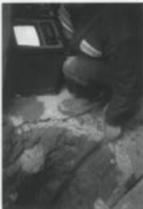
Fig. 16. Contractors specializing in building diagnostics often have video cameras or fiber optic equipment that allow the viewing of inaccessible areas. This is particularly helpful in chimney flues or subsurface drains, as shown here. In the past, these areas would need to be excavated for visual inspection. Photo: Austin.
