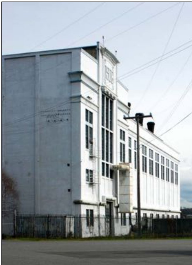
Figure 49: Northwest corner of the Steam Plant, with a view of the west façade and a portion of the north façade.
